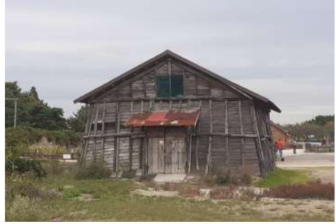
▲ Old salt warehouse of Sorae Salt Pond (Source: Korea Heritage Service)
