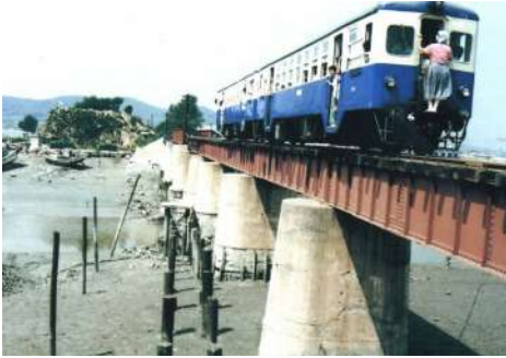
▲ Sorae Railway Bridge and train with narrow gauge (Source: Incheon Metropolitan City)
