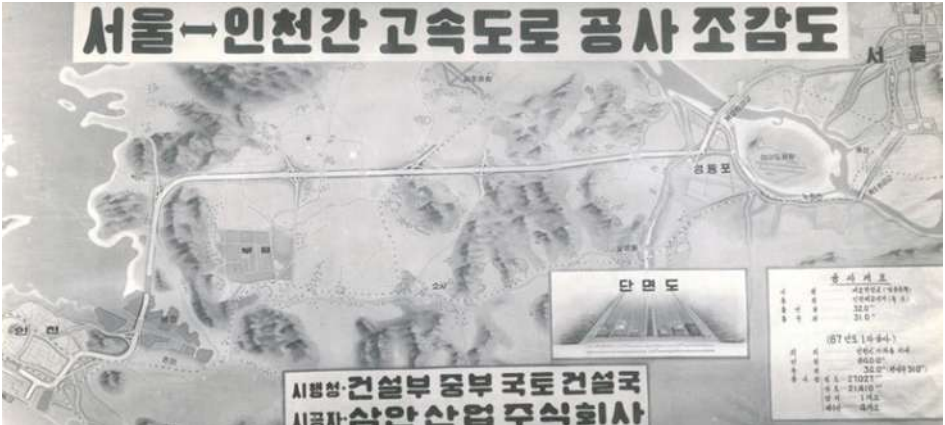
▲ Bird's-eye view of Gyeongin Expressway's construction (Source: Incheon Metropolitan City)
