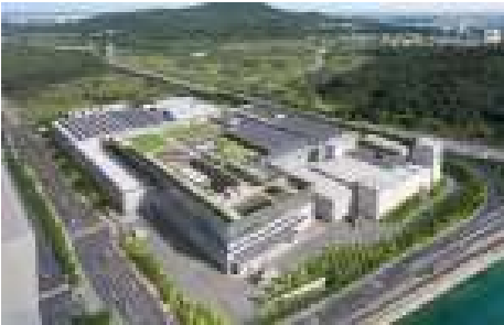
▲ Yeongjongdo Island Korean Air New Engine Repair Factory (Source: Incheon Metropolitan City)
