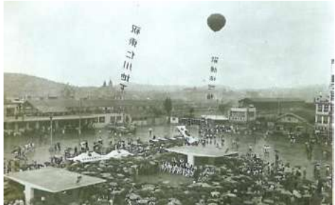
▲ Commencement of Dongincheon Underground Passage in 1967 (Source: 《History of Incheon Metropolitan City in Photos vol. 2》)
